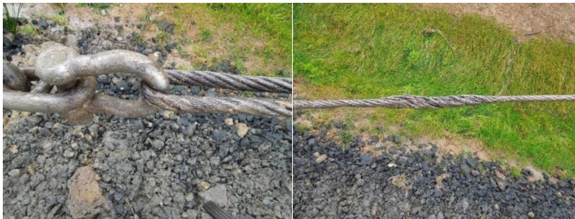
Figure 5: Spliced eye end connection and splice of system 4
