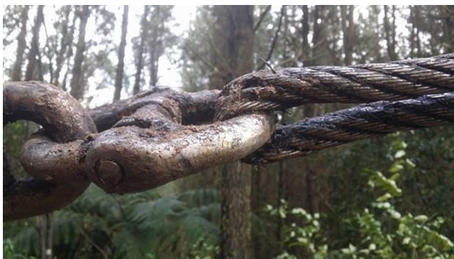
Figure 2: Spliced eye rope end connection used by system 1
