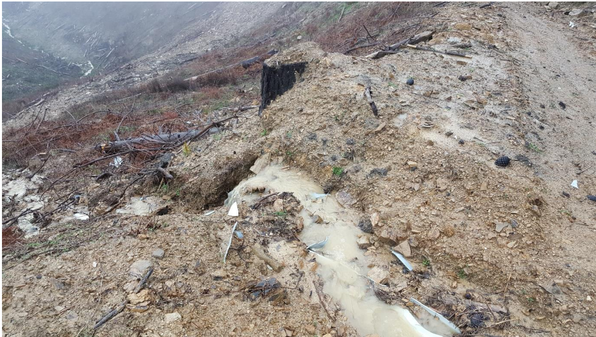
Figure 3. Dysfunctional cut-out and consequential runoff
