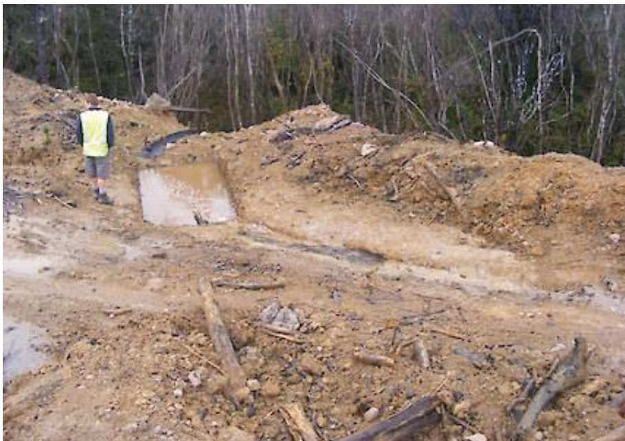
Figure 5. Photo of sediment trap installed to reduce the amount of coarse sediment in runoff before its discharged via flume (from NZFREM)
