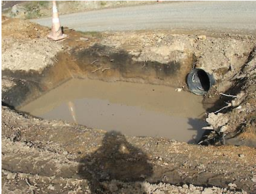
Figure 6. Photo of soak hole. There is only inlet, because sediment laden water will be soaked into porous soil (from NZFREM)
