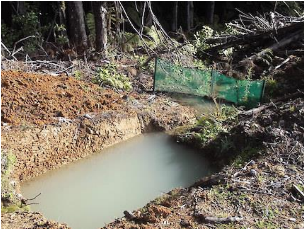
Figure 7. Sediment trap and Silt fence together (retrieved from NZFREM and ESGFO)
