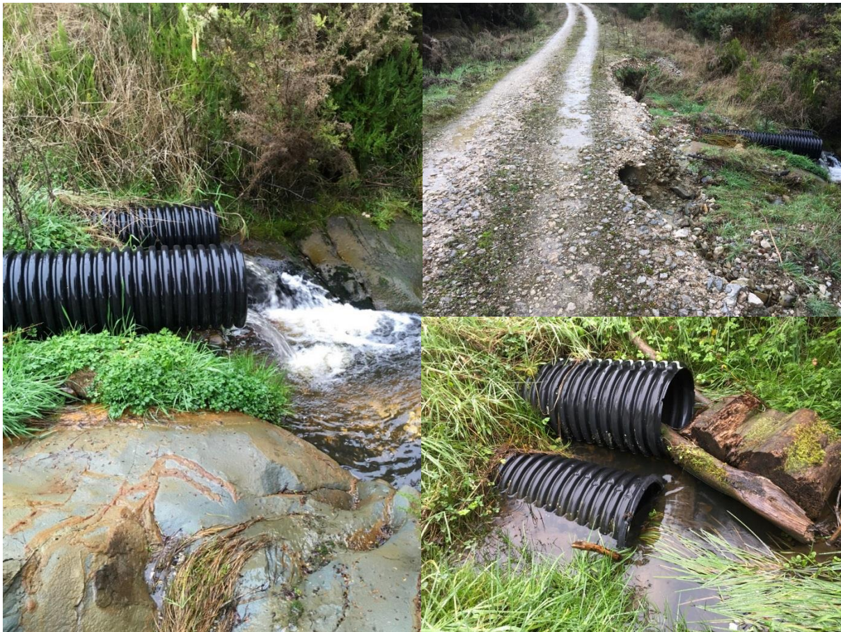
Figure 21- Inlet of these 2 plastic pipes are blocked with woody debris do not appear to sit in a defined stream channel. The road has been eroded away when this crossing floods. The outlets are also perched and have an overhang.
