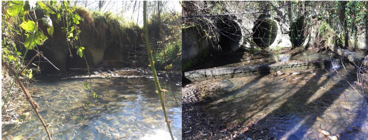
Figure 21- This large concrete crossing with 3 pipes has an apron with a small perch on the outlet this perch could be quickly built up with a rock ramp.
