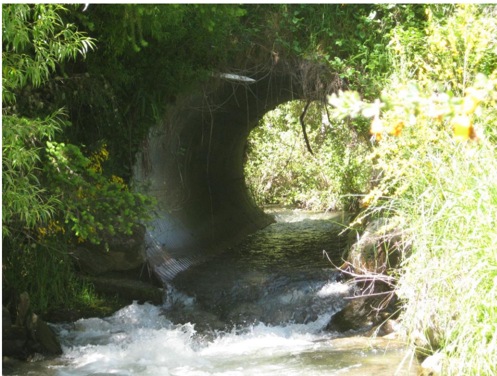
Figure 8- Large corrugated iron culvert with a medium perch, has had remediations which have washed away due to the high velocity of water.
