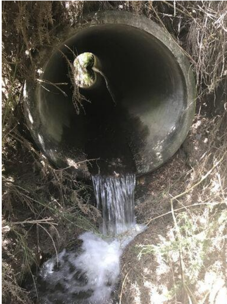
Figure 12- this medium size concrete culvert has a small perch and overhang. It was easily remediated through the installation of a fish mat and Spat ropes.
