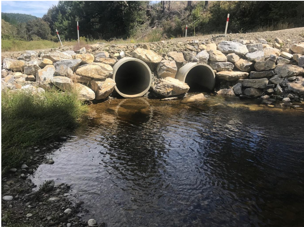
Figure 13- Newly installed concrete 2 pipe crossing. Second pipe is lower to aid fish passage
