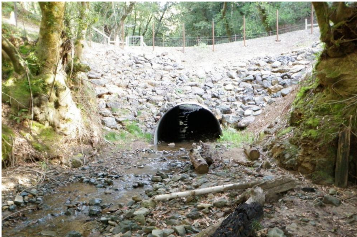
Figure 1- Correctly inverted culvert (Pacific Watershed, 2018)
