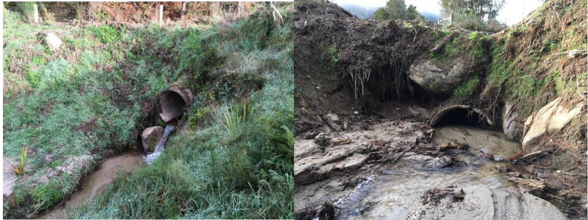
Figure 20- Single concrete culvert has large silt build up at inlet and large perch and overhang at outlet. Outlet is good for fish mat and spat ropes.
