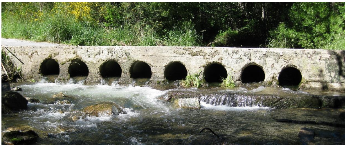
Figure 17- This concrete splash culvert with 8 pipes regularly blocks in flood events. It also has a high velocity which is increased by the lack of friction in the concrete pipes. Could be fixed through replacement or slowing the velocity in one pipe to aid fish passage.
