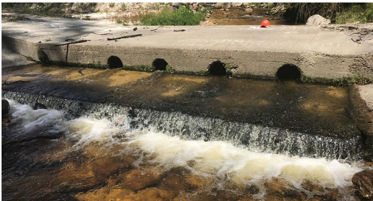
Figure 14- 4 pipe concrete splash culvert, apron slows velocity, but, creates small perch which has been remediated through creating a rock ramp at one end
