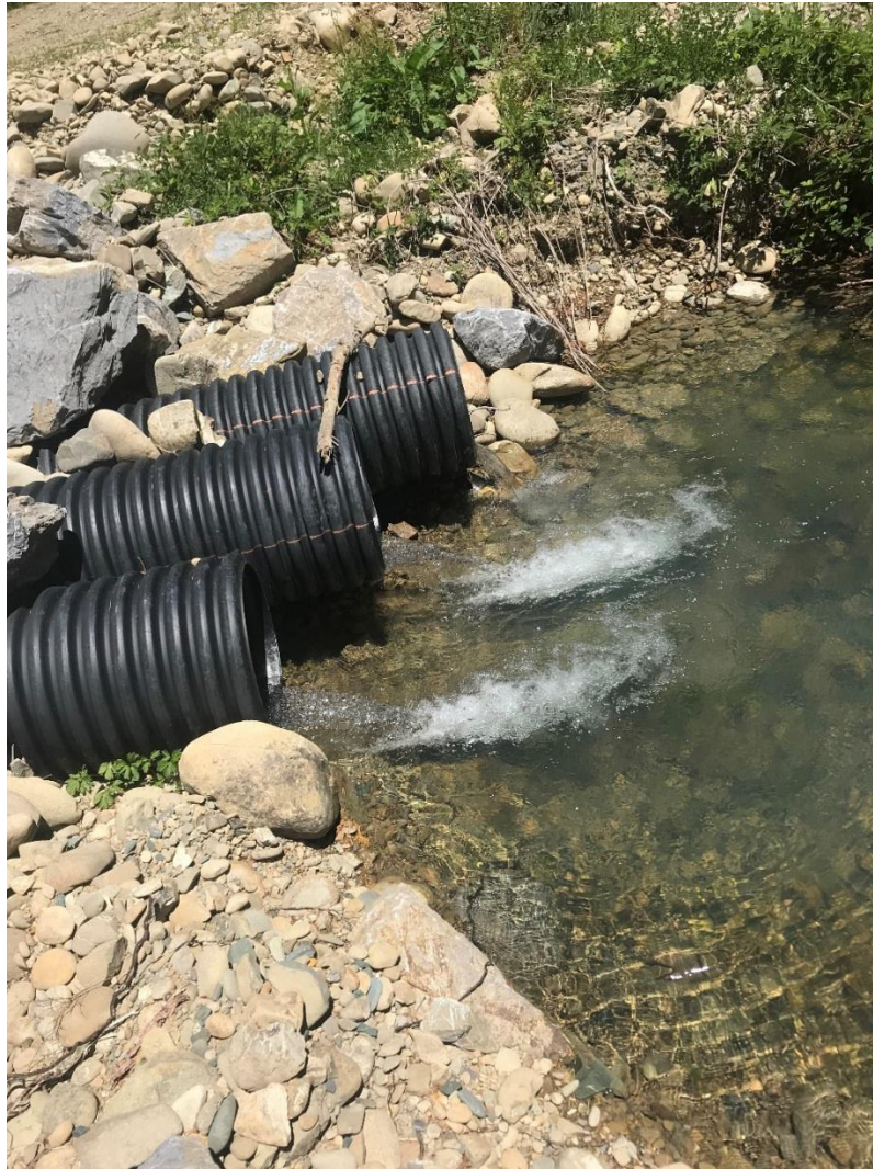
Figure 18- These three plastic pipes were a temporary culvert and have now been removed. Their passage issue is that they are perched with an overhang.
