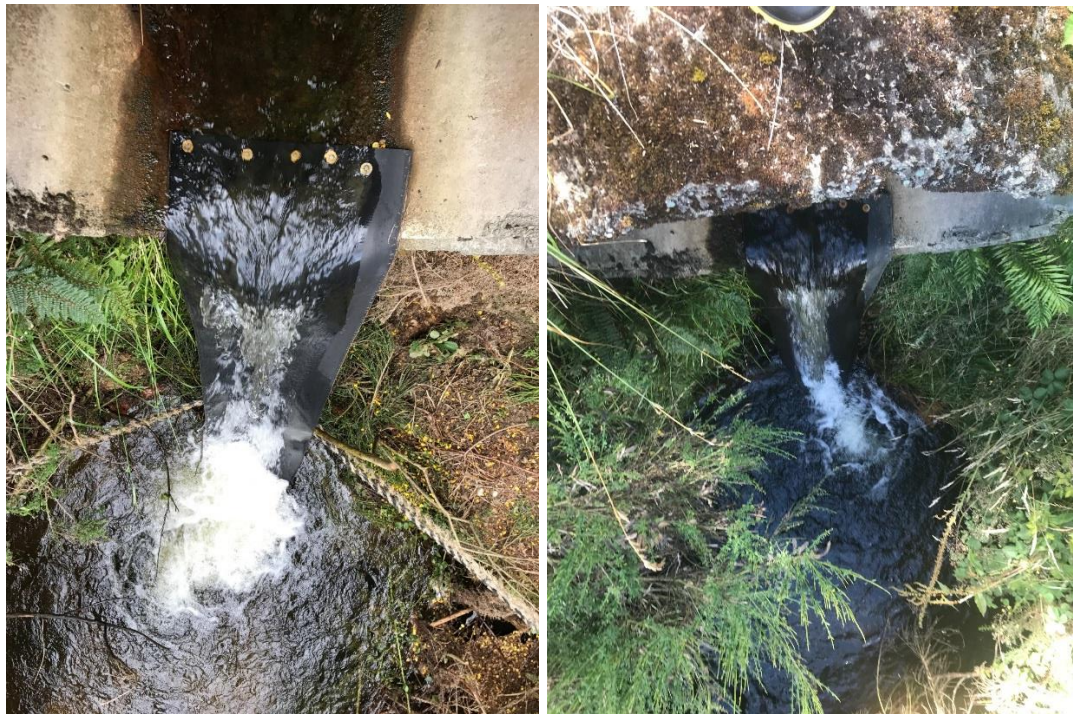
Figure 6- Aerial view of fish mat set up over a 3m perch
