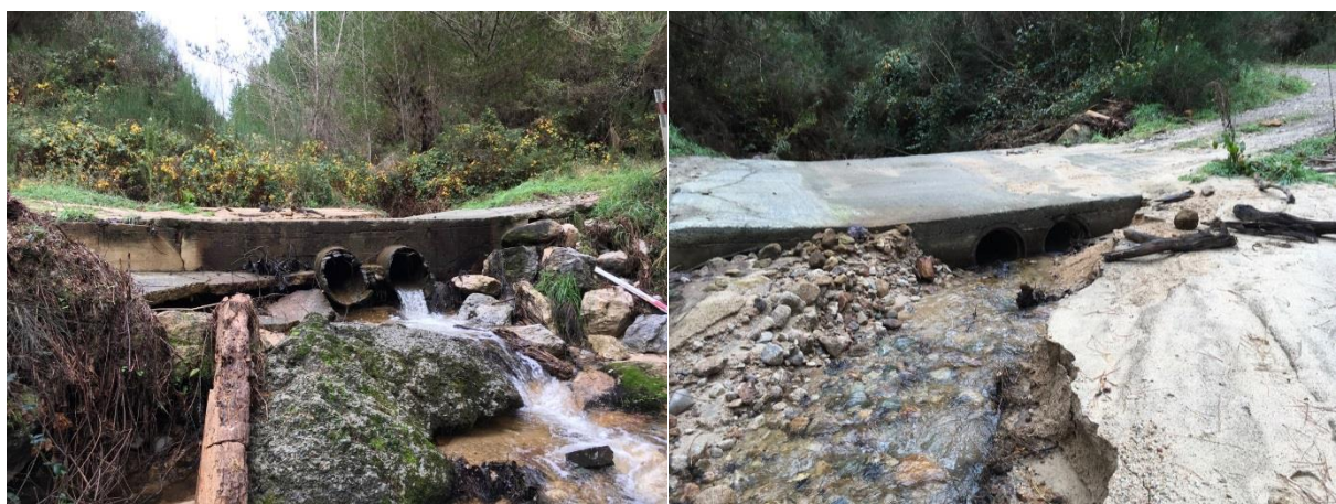
Figure 19- This crossing is a concrete splash with 2 pipes. It has been damaged and has a large overhang, perch and velocity in 1 pipe while the other is blocked by a silt build up. This needs to be pulled out and replaced with a culvert designed for greater capacity.
