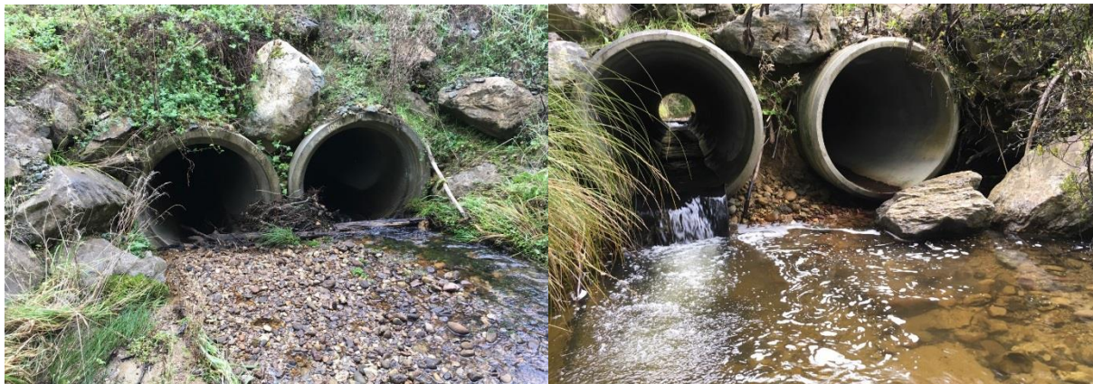
Figure 23- This double concrete culvert is perched and overhung. It has already been remediated with a fish mat.
