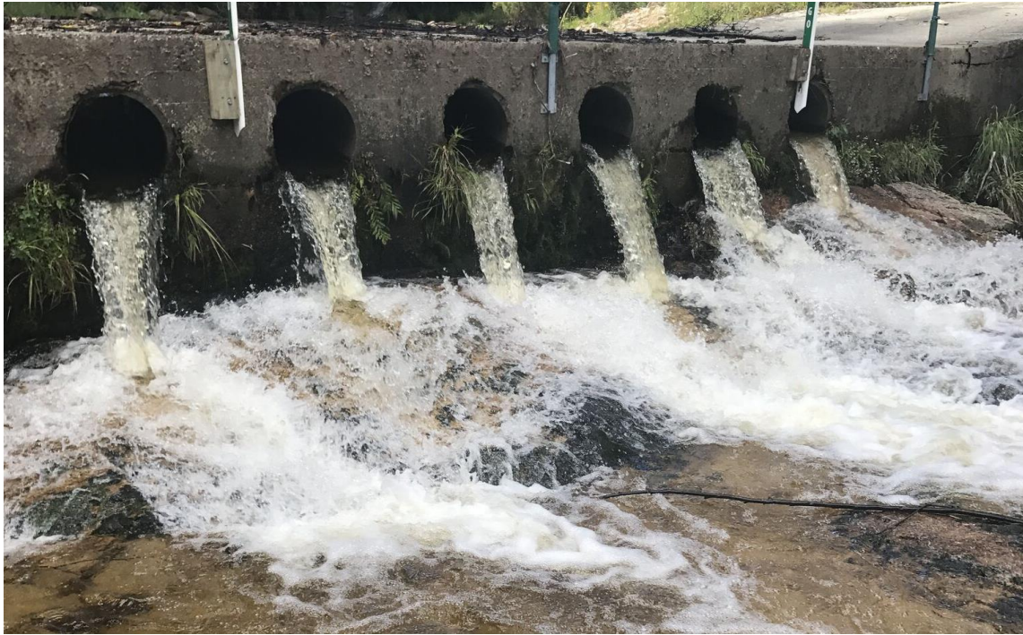
Figure 9- 6 pipe concrete splash culvert, high velocity 0.3-0.5m perch and large sediment build-up upstream. Has now been replaced with bridge due to the large sediment build ups and regular flooding of this crossing
