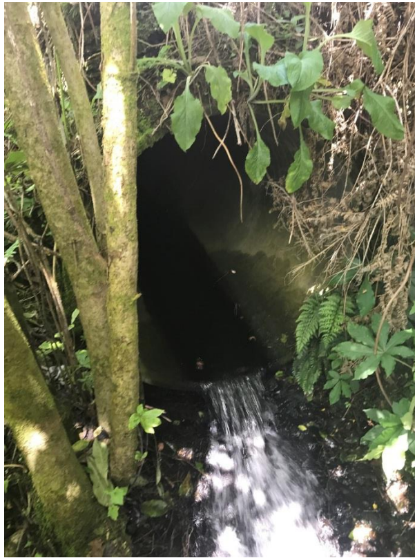
Figure 16- This medium size concrete culvert has a small perch and overhang. It was easily remediated through the installation of a fish mat and Spat ropes.
