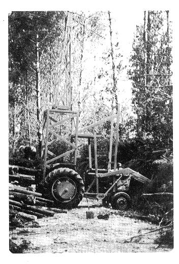
For thinning, if the piece size is right, and more importantly if there is a market for the wood, small haulers like this are both practical and economic. The basic unit is a farm tractor, with an Igland double-drum winch driven from the P.T.O. of the tractor. There is provision to run both a skyline and strawline through drums bolted on to the rear wheels of the tractor. The tower is built locally and the all-up cost of the unit is \$20,000-\$25,000.
