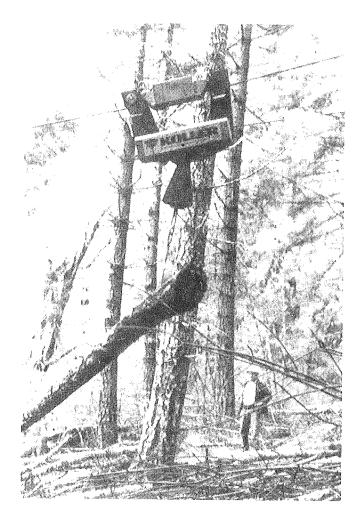
A step up in complexity is hydraulically activated locking carriages like the Koller and Wyssen. Because of their internal mechanisms, the manufacturer recommends load limits for each size of carriage. For example, this Koller carriage has a load limit of 2.5 tonnes.
