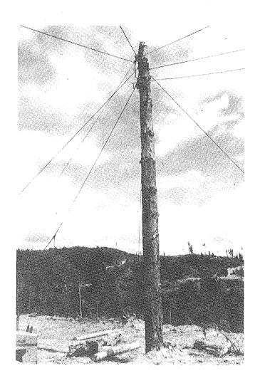
All of the haulers you've seen so far are rigged through a standing tree. There's nothing wrong with this, but I suspect that the expertise to rig correctly and safely will be somewhat lacking in crews working a limited scale.
