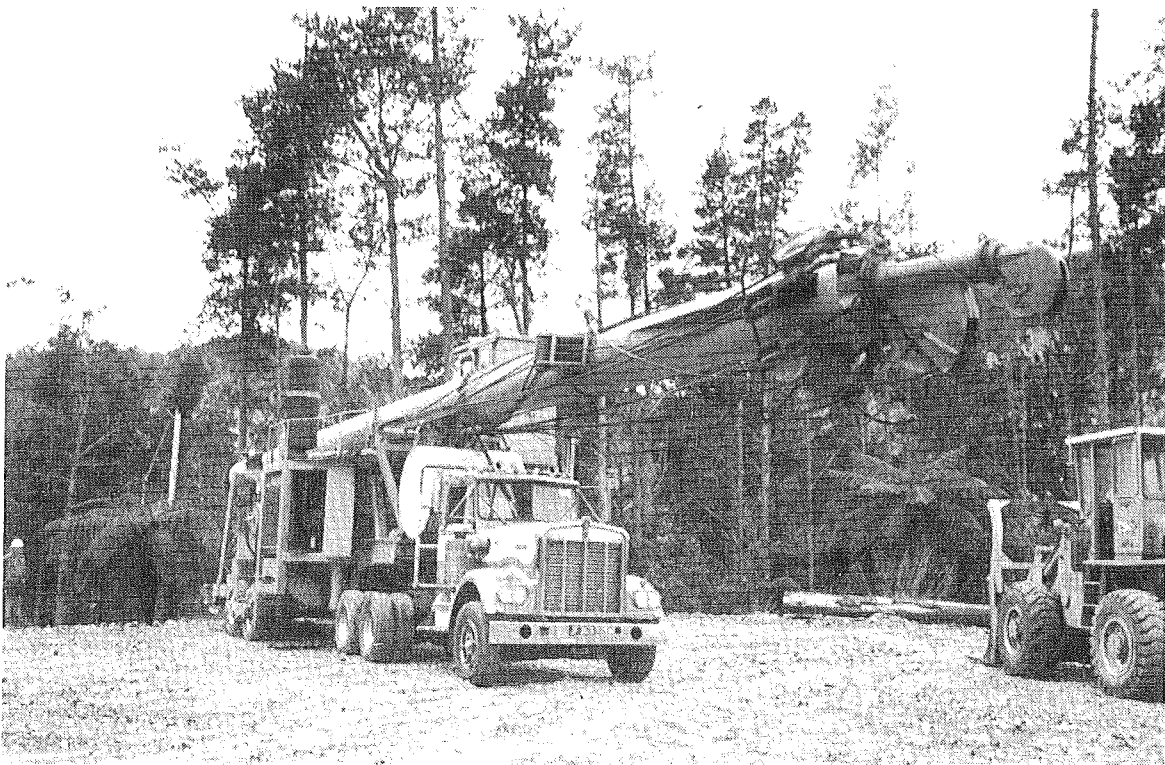
Trailer-mounted Skagit spar being manoeuvred into position on a new landing by a transporting truck.
