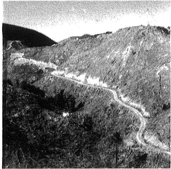
Figure 6 - End hauling to reduce visual impacts and excessive erosion.
