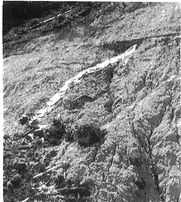
Figure 5 - Using a culvert "sock" to divert water past the fill slope.
