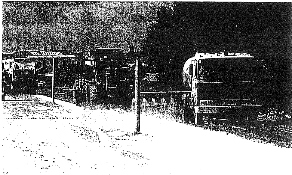
Fig 1 Lime slaked from side shift boom
