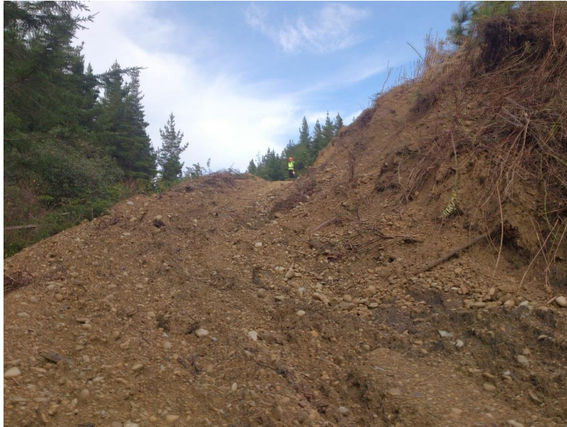
Figure 8. This temporary stream crossing approach was steep (33% slope), with no water control, and poor surface cover (20% cover). The potential erosion rate was estimated at 204 tonnes/hectare/year.
