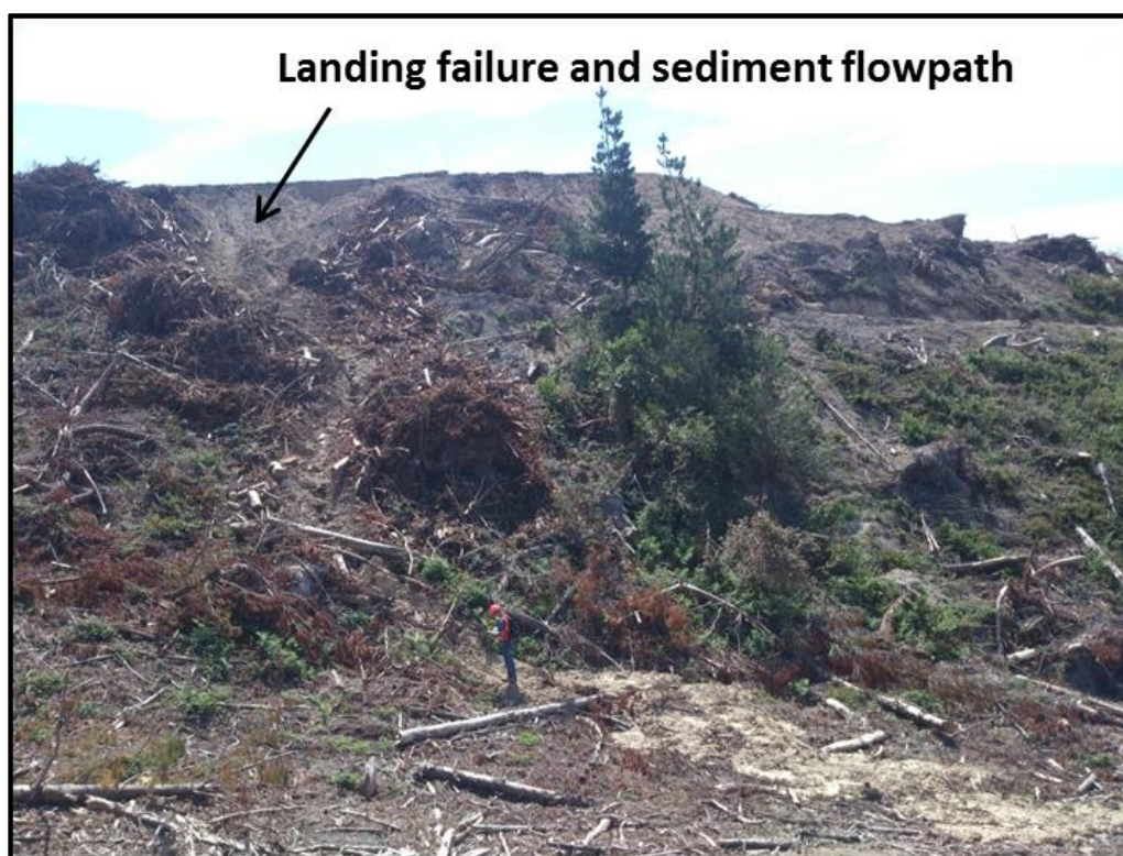
Figure 1. Example of a sediment breakthrough to an ephemeral stream channel. This breakthrough resulted from a landing failure. Photo: Kristopher Brown.
