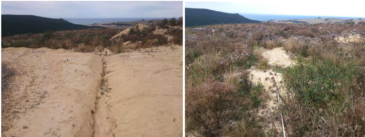
Figure 5. Left: At a road curve, a cut-out moves water from the ditch into an area in the cut-over with flat topography and high surface roughness, ideal for trapping sediment. Right: Sediment is trapped and stored in the cut-over.
