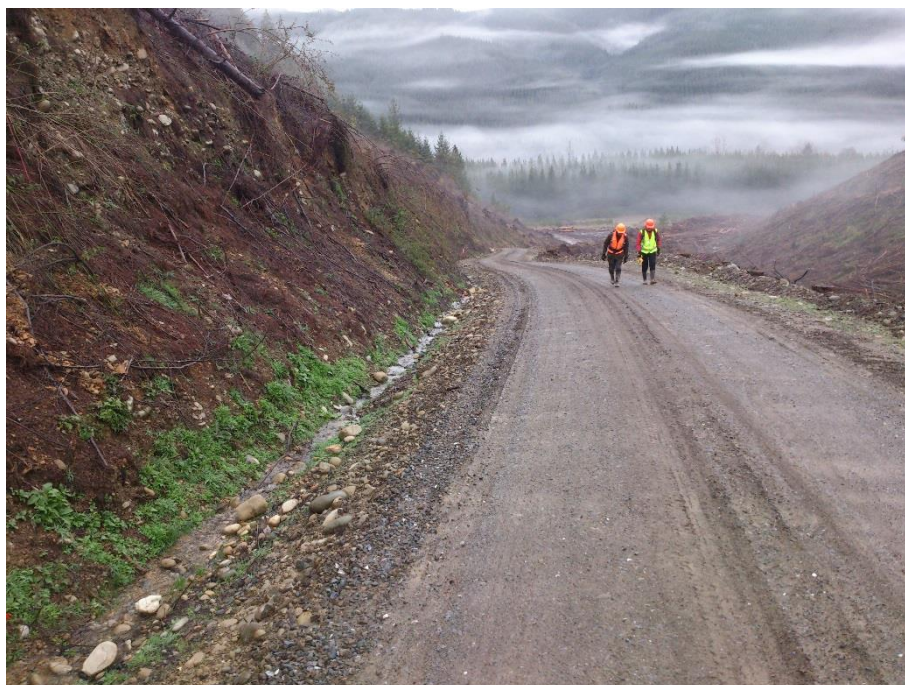
Figure 6. A secondary forest road with a good shape (crown), which moves half of the road surface runoff to the inside ditch and half to the fillslope (outer) side of the road. Water in the ditch drains to a series of cross-drain culverts, while surface runoff from the outer half of the road is relieved by a series of cut-outs. Note that the ditch also concentrates subsurface flow
