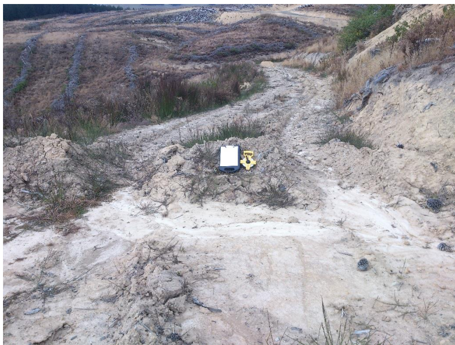
Figure 10. Surface runoff passes through this water bar because it has been compromised by traffic.
