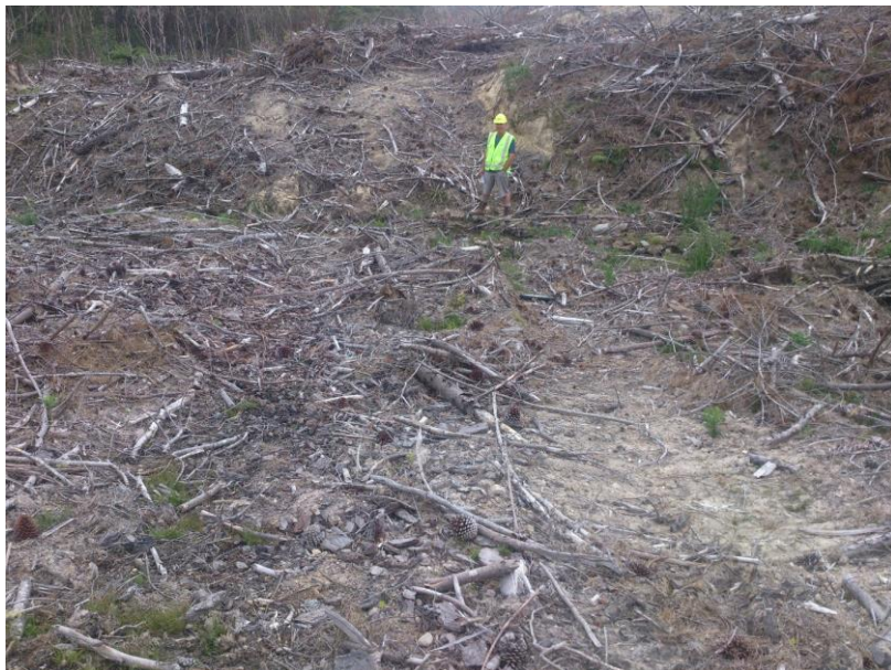
Figure 9. This temporary crossing has gentle approaches to the stream, slash barriers were used to disrupt concentrated surface runoff, and logging slash was used to provide surface cover.
