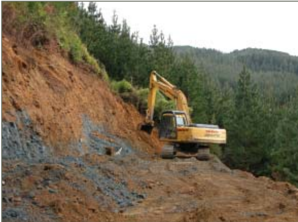
A good example of excavator construction of a mid slope road using balanced cut and fill.
