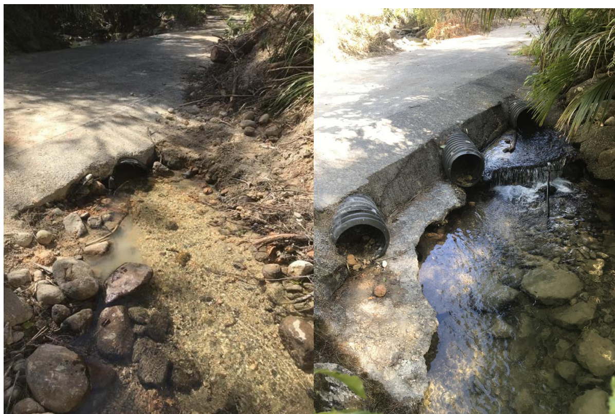
Figure 4.6 Showing RMFID67 a battery culvert crossing with upstream on the left and downstream on the right.
