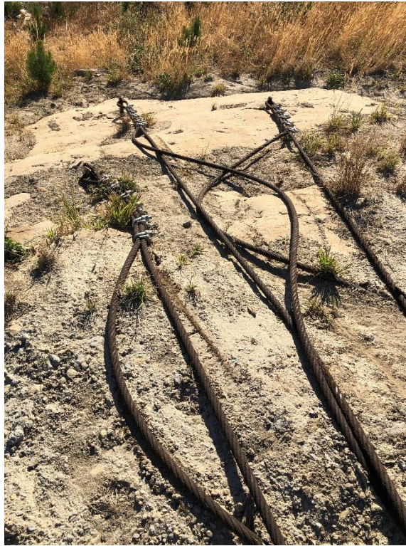
Figure 21 - Imbalance in the rigging of the trio of grouted rock anchors
