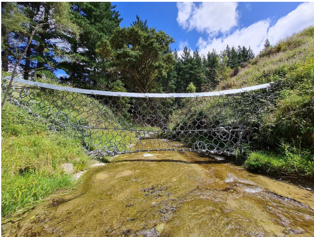
Figure 33 - Slash trap using grouted rock anchors as supports
