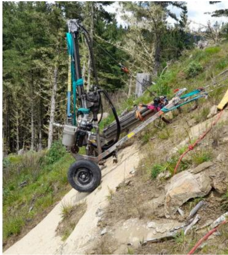
Figure 24 - Pneumatic drilling rig used in the installation process
