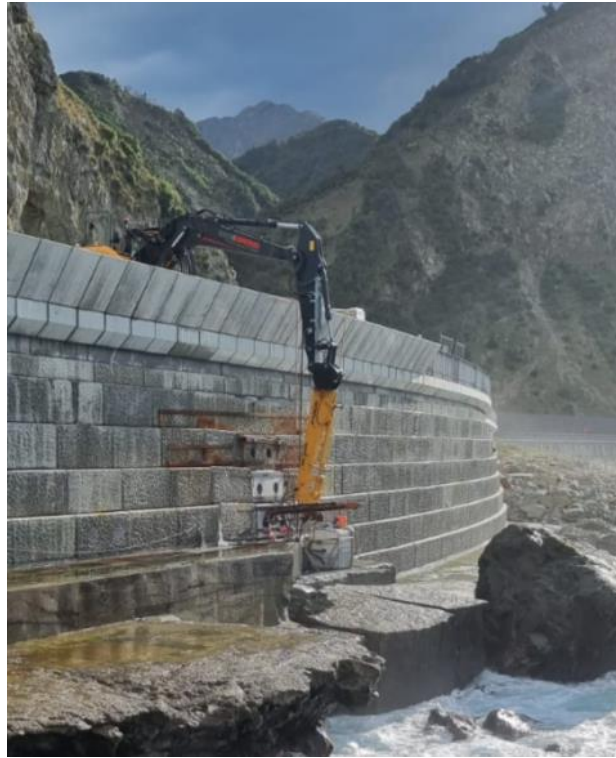
Figure 25 - Example of excavator-based drilling rig
