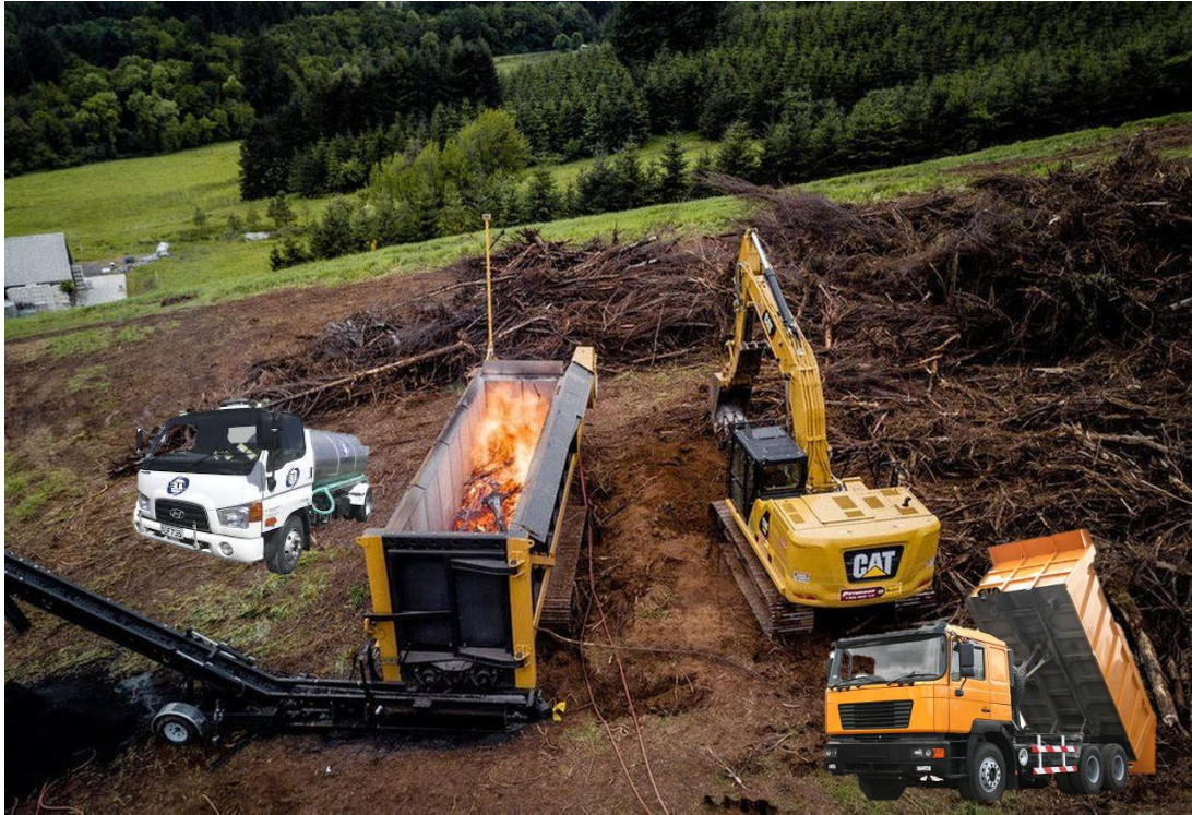
Figure 11. Carbonator operation supported by 2 x crew, 14T digger, 5000L water truck and a bulk truck.
