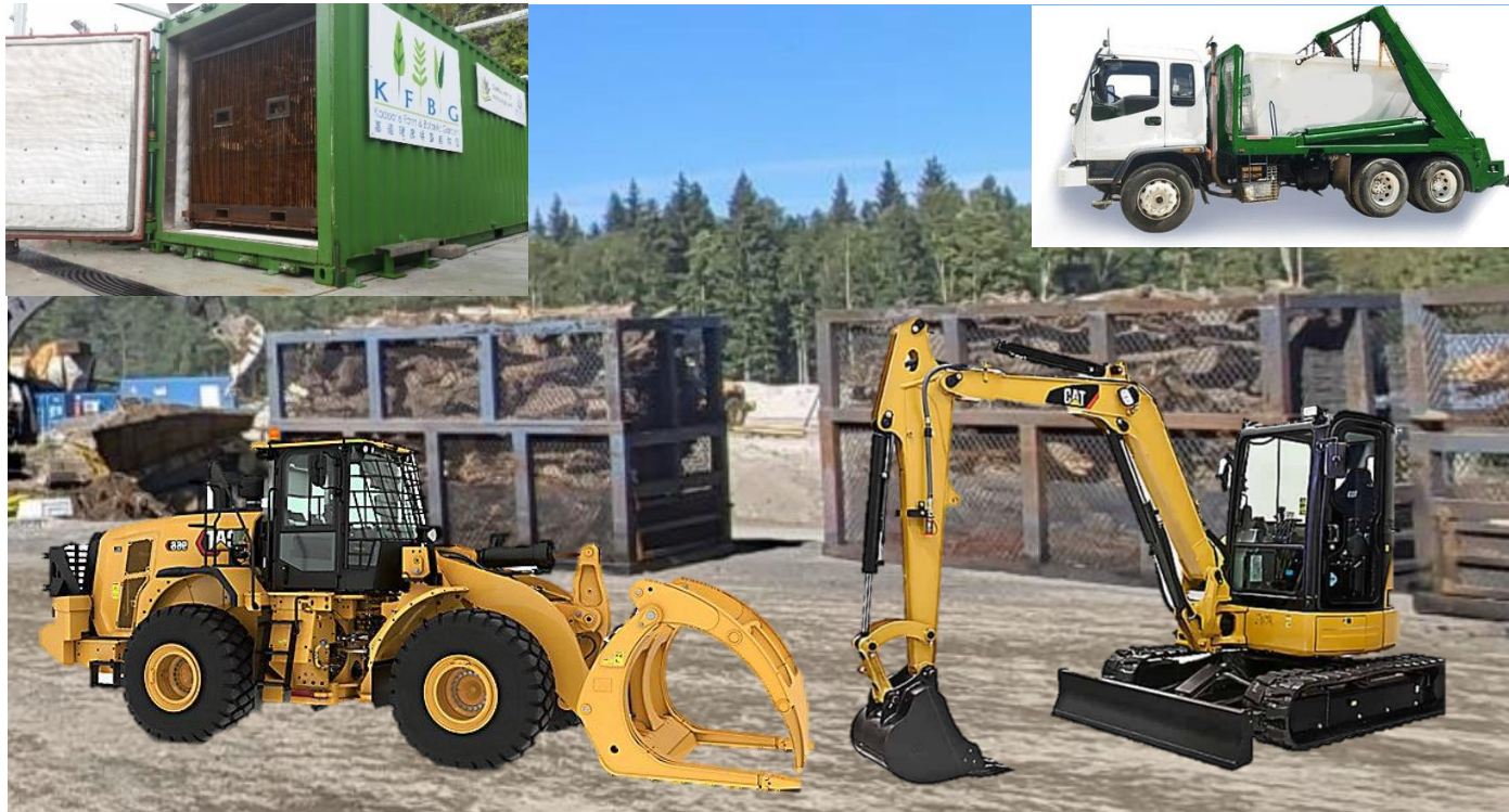
Figure 12. Charmaker operation supported by 1 x crew, 20T front end loader, 5.5T digger, 15m 3 skip with truck.
