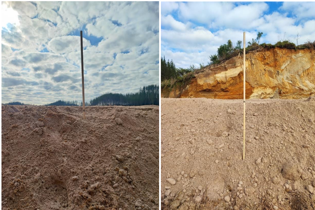
Figure 31 & 32: Image displaying how desired 750mm layer thickness was achieved.
