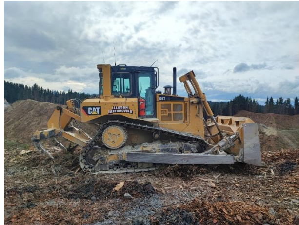
Figure 14: CAT D6T which was used for compaction at site 1.
