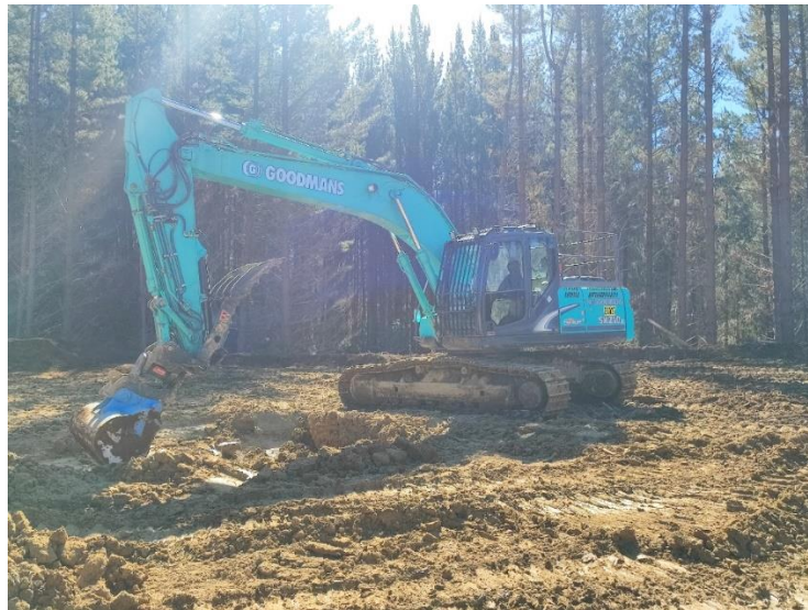
Figure 24: Kobelco SK210LC excavator
