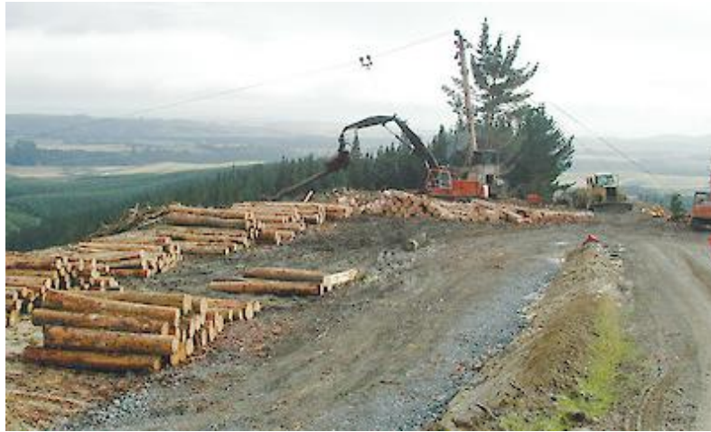
Figure 3. – An example of a spur road end landing configuration taken from FOA (2020).
