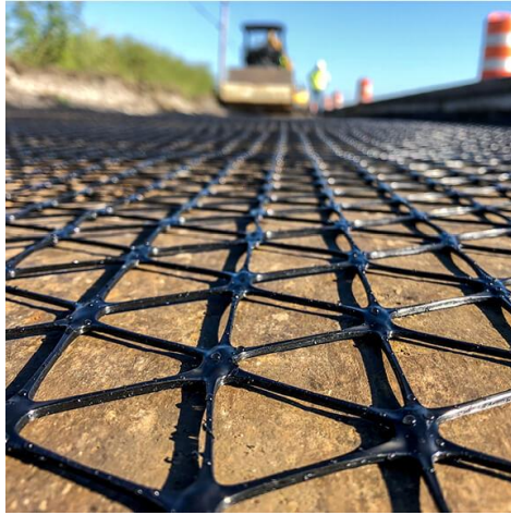
Figure 11: Triaxial geogrid laid over a road subgrade (Tensar International Corporation, 2021).
