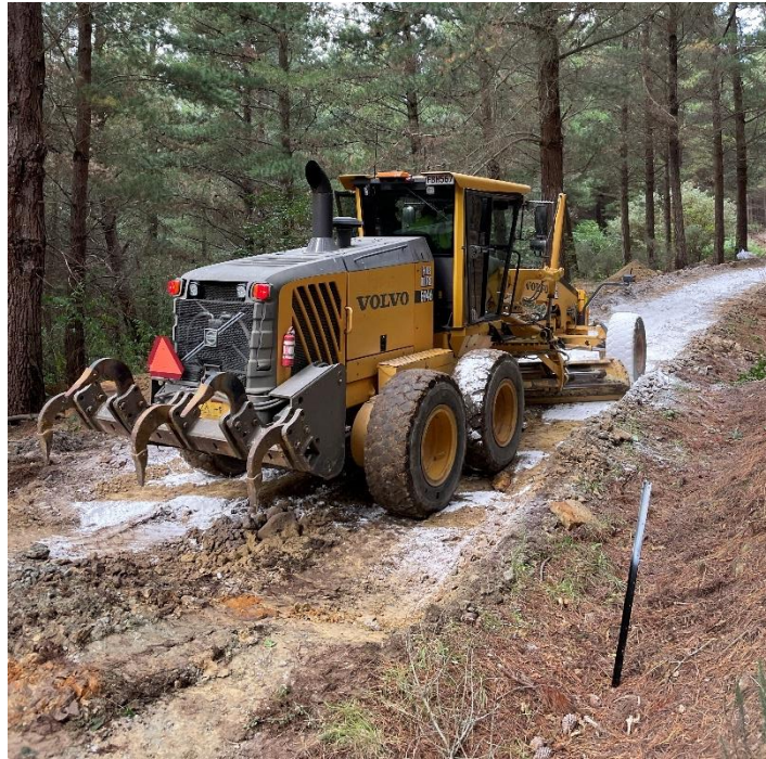
Figure 18: Grader beginning to mix lime through Diamond Hill Road.
