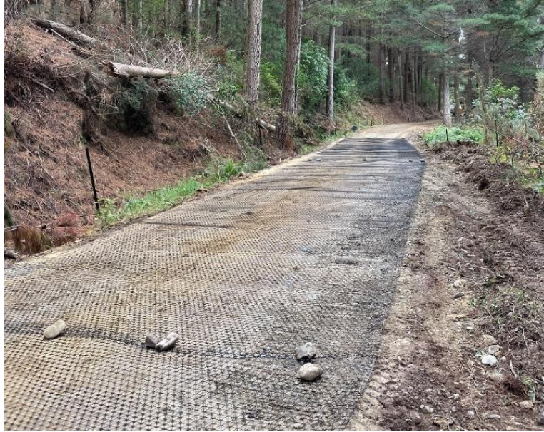
Figure 17: Installation of geogrid on Diamond Hill Road.
