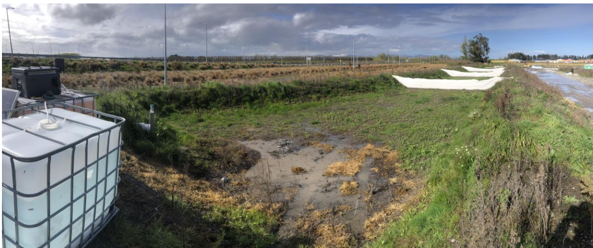
Figure 16: Empty sediment retention basin used for the in-situ testing.
